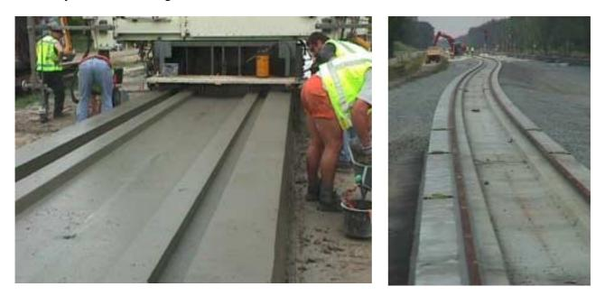
Figure 2 Construction of Embedded Rail with paver (Test track near Best, the Netherlands; source: Strukton Railinfra)
